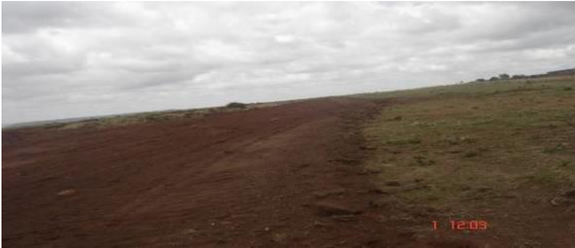
Figure: 4.20. Top soil is reinstated to speed re-growth of vegetation in the area. A visual inspection needs to be conducted at least bi-annually to monitor re-growth of this borrow pit site.
