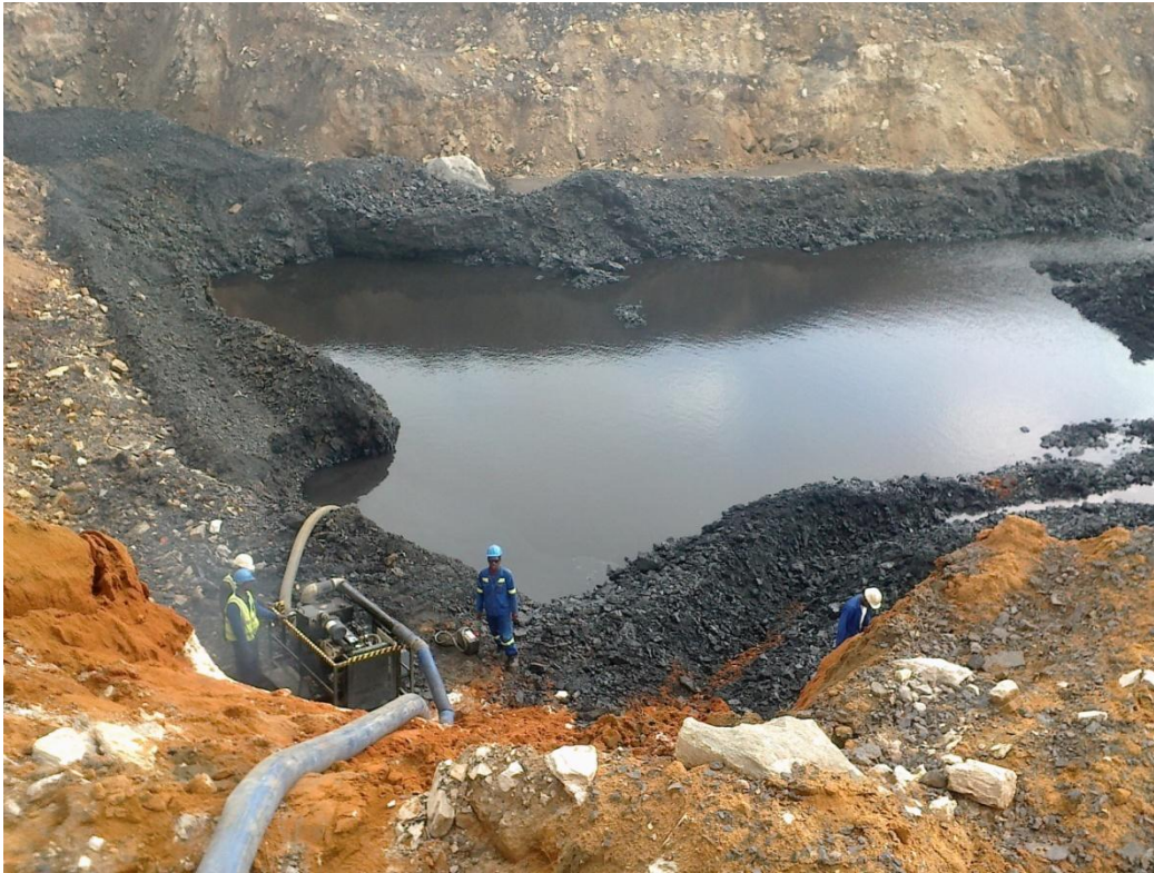
Figure 4.6: Water being pumped out of the pit
