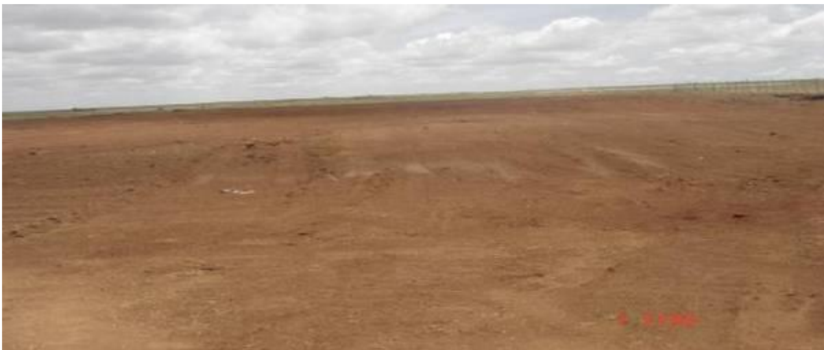
Figure: 4.19. Reshaping of this borrow pit land was blended into the surrounding landscape to reduce the likelihood of erosion. This allows for natural drainage patterns to be re-established.
