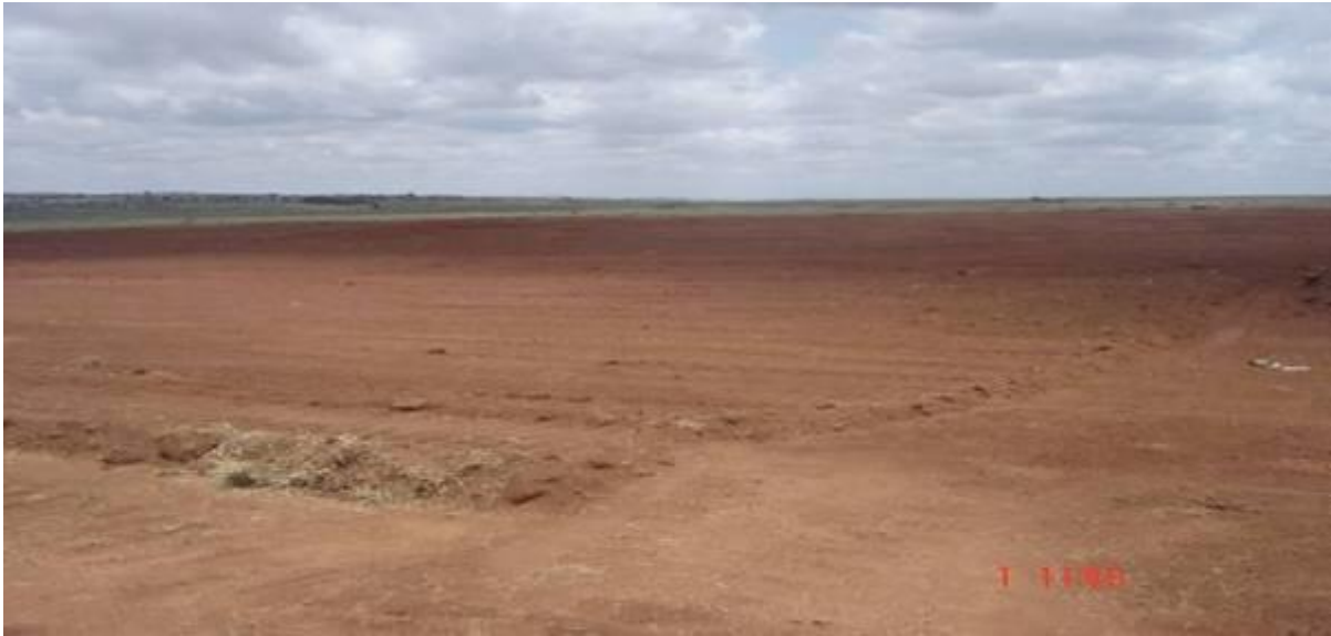
Figure: 4.18. This picture shows that the borrow pit area is backfilled with extra materials to eliminate the depth thereof.
