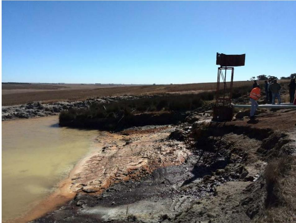
Figure 1.3: AMD decant from closed mine workings in quaternary catchment X11B, near Carolina. The decant had occurred once the mining operation had been seized, and during the plans to rehabilitate the land, the mining company who owned the rights to the land filed for liquidation, which is discussed later on in this work.
