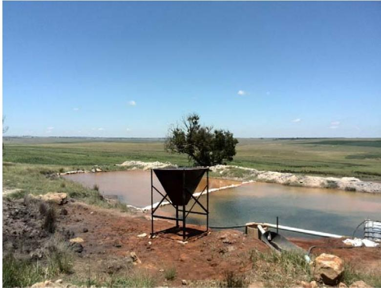
Figure 1.5: Lime being used as a temporary treatment for AMD decant in Carolina. This was a plan put in place while the mining company and regulators discussed long term solutions to the decant at the seized mining operation.
