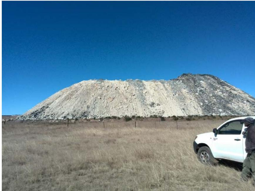
Figure 4.8: A typical mine dump of overburden in quaternary catchment X11B.
