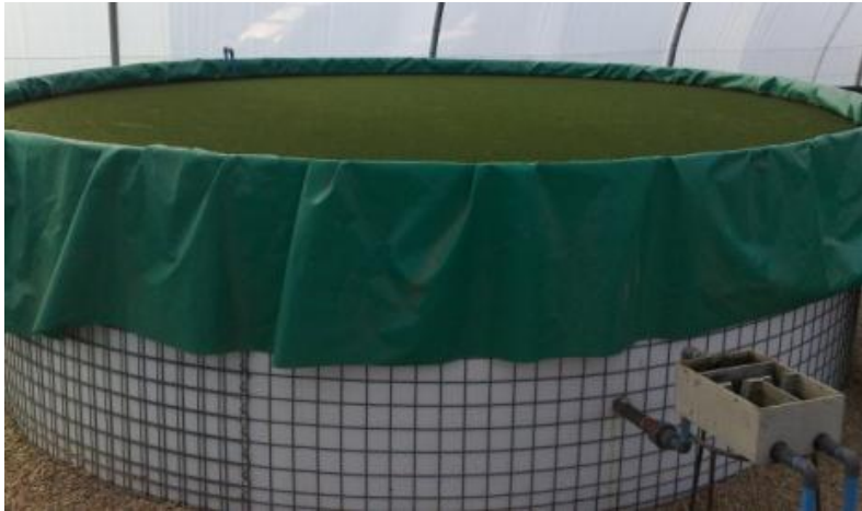
Figure 2.1: Primary facultative pond and splitter box.
