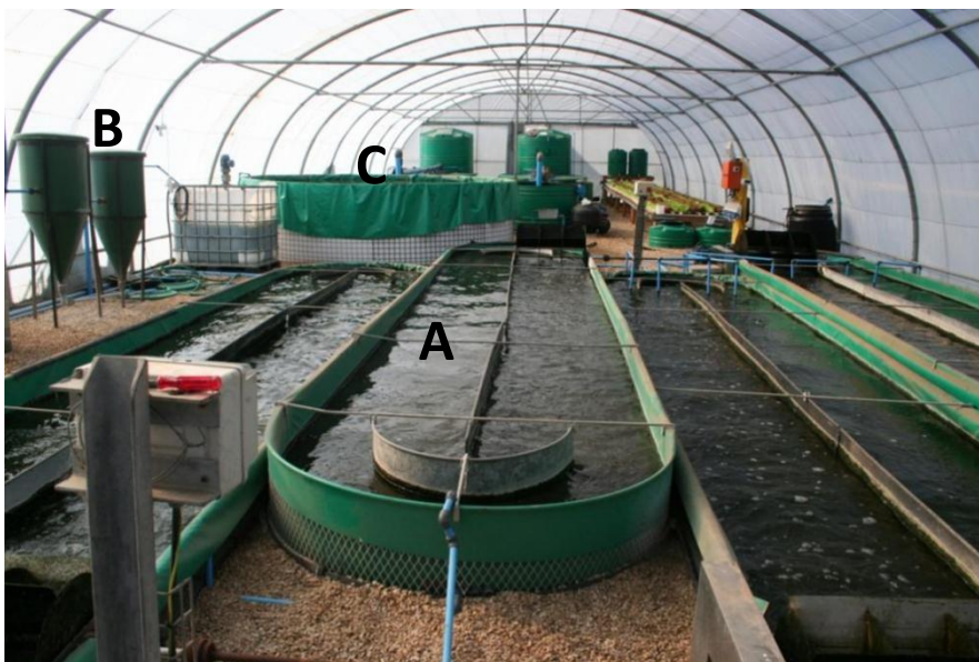
Figure 2.2: High rate algal ponds used to treat anaerobically digested brewery effluent in the foreground (A), with algal settling cones on the left (B) and the primary facultative pond in the centre (C).
