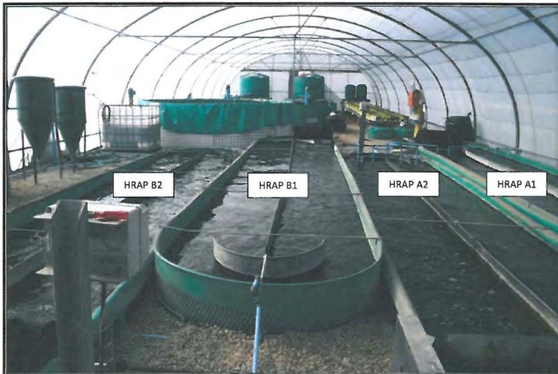
Figure 3.1.i: High rate algal ponds (HRAP) A1, A2, B1 and B2.
