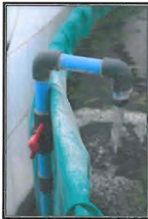
Figure 3.1.f: The inlet valve used to control the hydraulic retention time in the primary facultative pond and high rate algal ponds.
