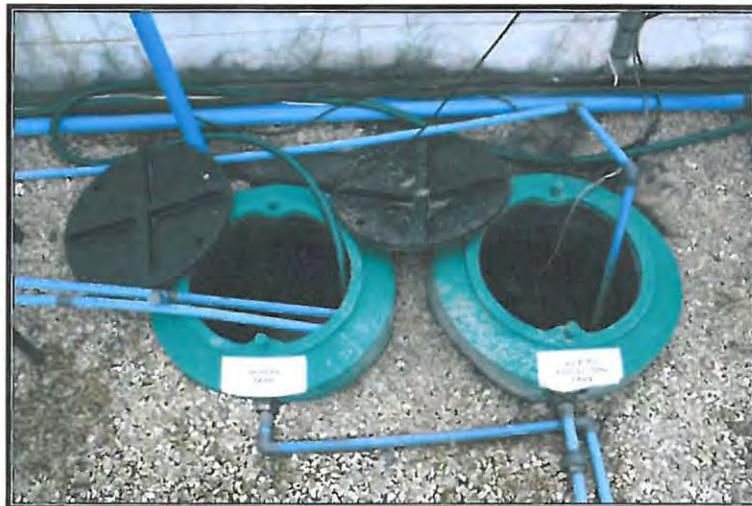
**Figure 3.1.l:** The submersed collection tank for high rate algal pond A2 and B2 effluent (right). The recessed slurry collection tank into which algae from harvesting tanks were drained weekly (left).
