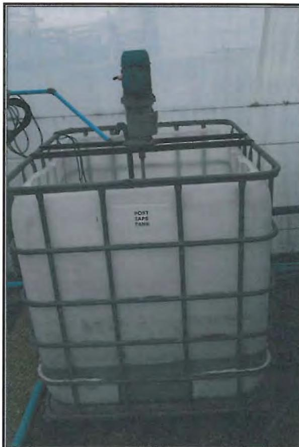
**Figure 3.1.n:** The 1000 L collection tank used to collect clarified high rate algal pond treated effluent.
