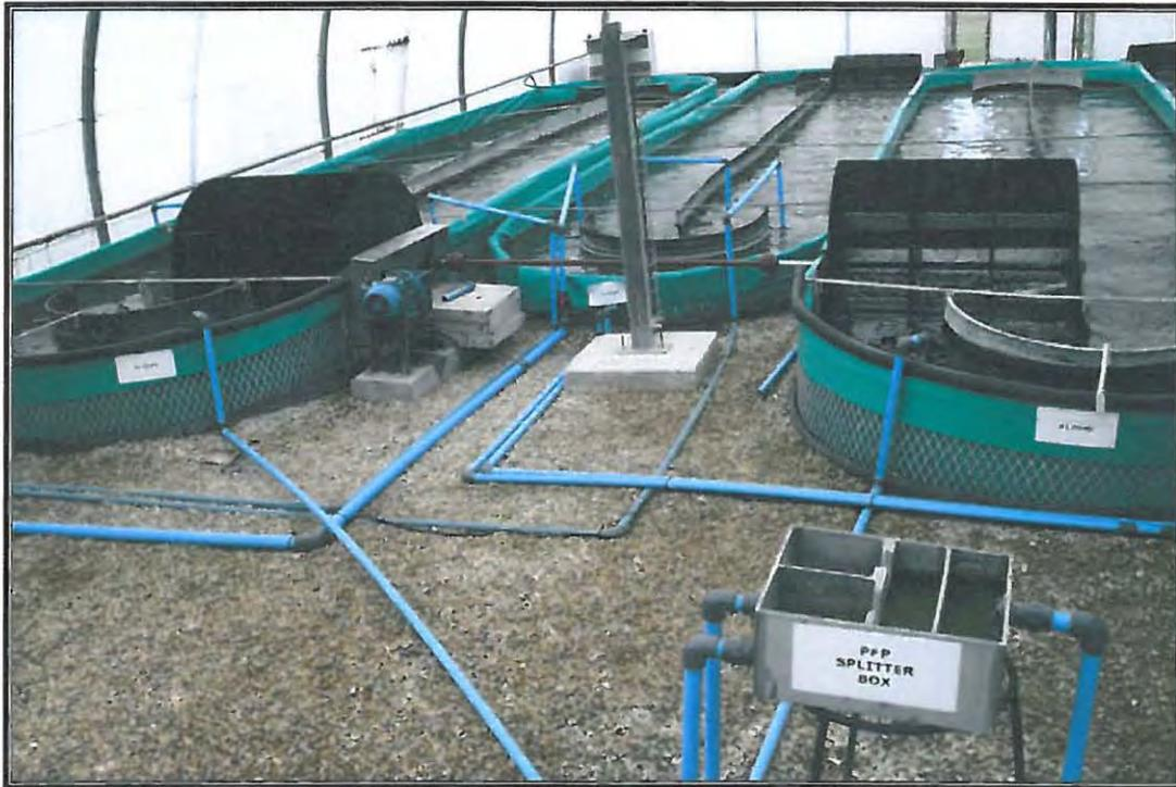
Figure 3.1.h: Effluent was diverted from the primary facultative pond into high rate algal ponds train-A and train-B.
