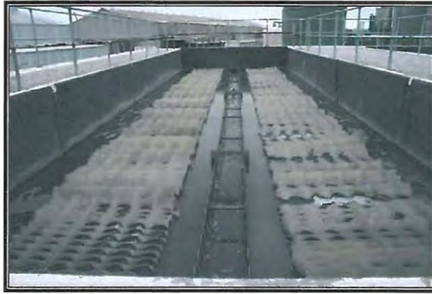
**Figure 3.1.b:** A view on top of the iBhayi brewery anaerobic digester.
