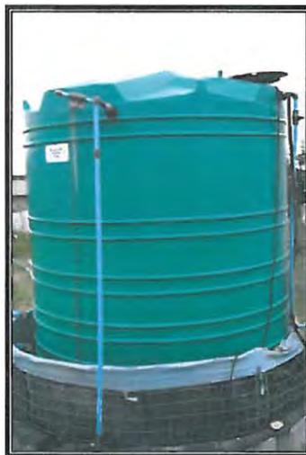
**Figure 3.1.d:** The pilot plant anaerobic digester.
