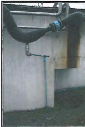
**Figure 3.1.c:** The connection point that diverted approximately 1 m<sup>3</sup>/d anaerobically digested effluent from the iBhayi brewery anaerobic digester into the pilot plant anaerobic digester.
