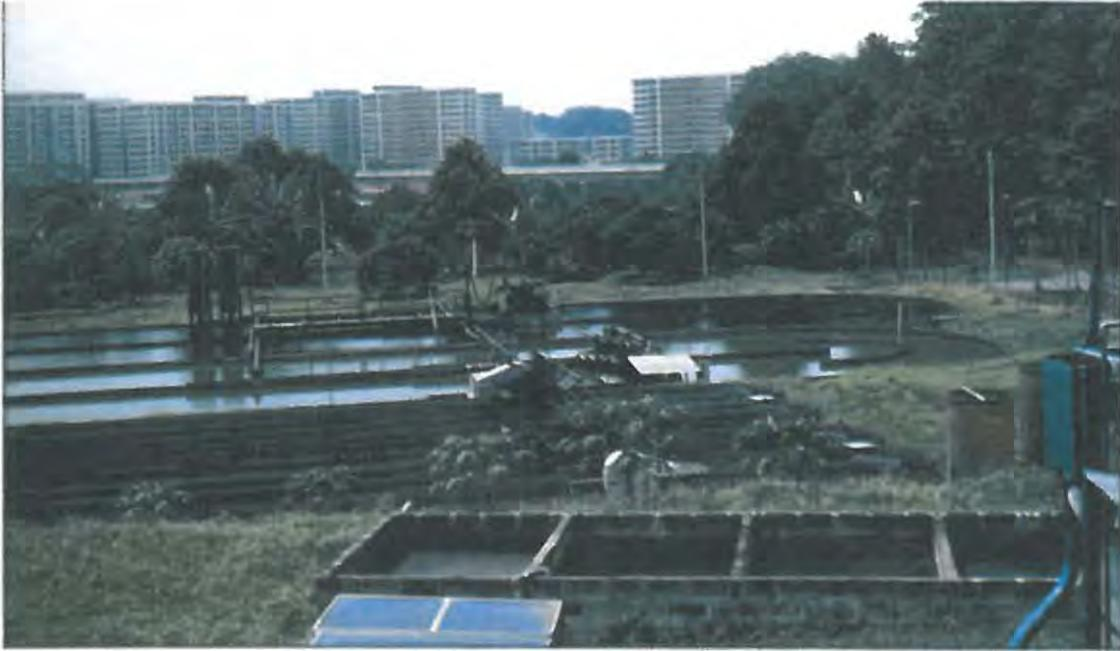
**Figure 2.3.2.a:** High rate algal ponds used in piggery effluent treatment (Singapore, Malaysia). Sedimentation tanks are in the foreground (Phang 1991).
