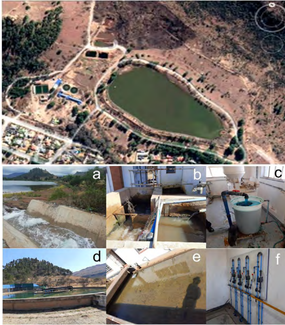
Figure 3.2 Google Earth image of Queenstown WTP adjacent to Berry Reservoir (top panel) and a collage illustrating the steps in the water treatment process (bottom panel). a) Water detained in Berry Reservoir; b) inlet and chlorination of water from Berry Reservoir; c) aluminium sulphate/alum coagulant/flocculent treatment; d) clarification in Dortmund settlers; and, e) final chlorination of the top-flow prior to release to municipal reticulation.
