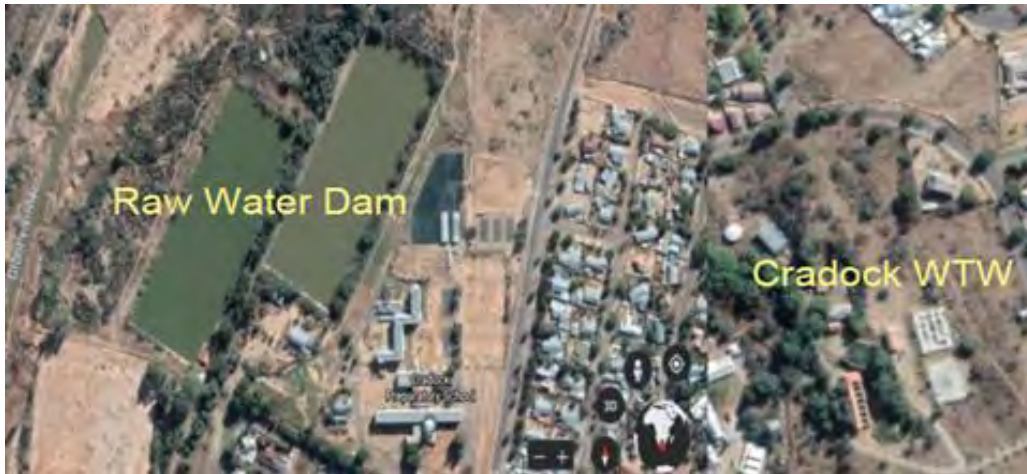
Figure 3.4 Raw water dams that store water from Gariep Fish-Sundays River Canal Scheme before it is channelled to Cradock WTP for treatment and reticulation to Cradock town.
