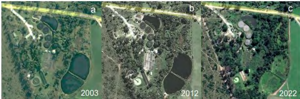
Figure 1.17 Apparent demise of process operations at the Belmont Valley WWTW from 2003 to 2022. In particular, changes to maturation dams from 2003 (a), 2012 (b) to 2022 (c). Overgrowth of the sludge drying beds; sludge accumulation in the primary settler; and dryness of biofilters, indicate a derelict and/or dysfunctional WWTW.
