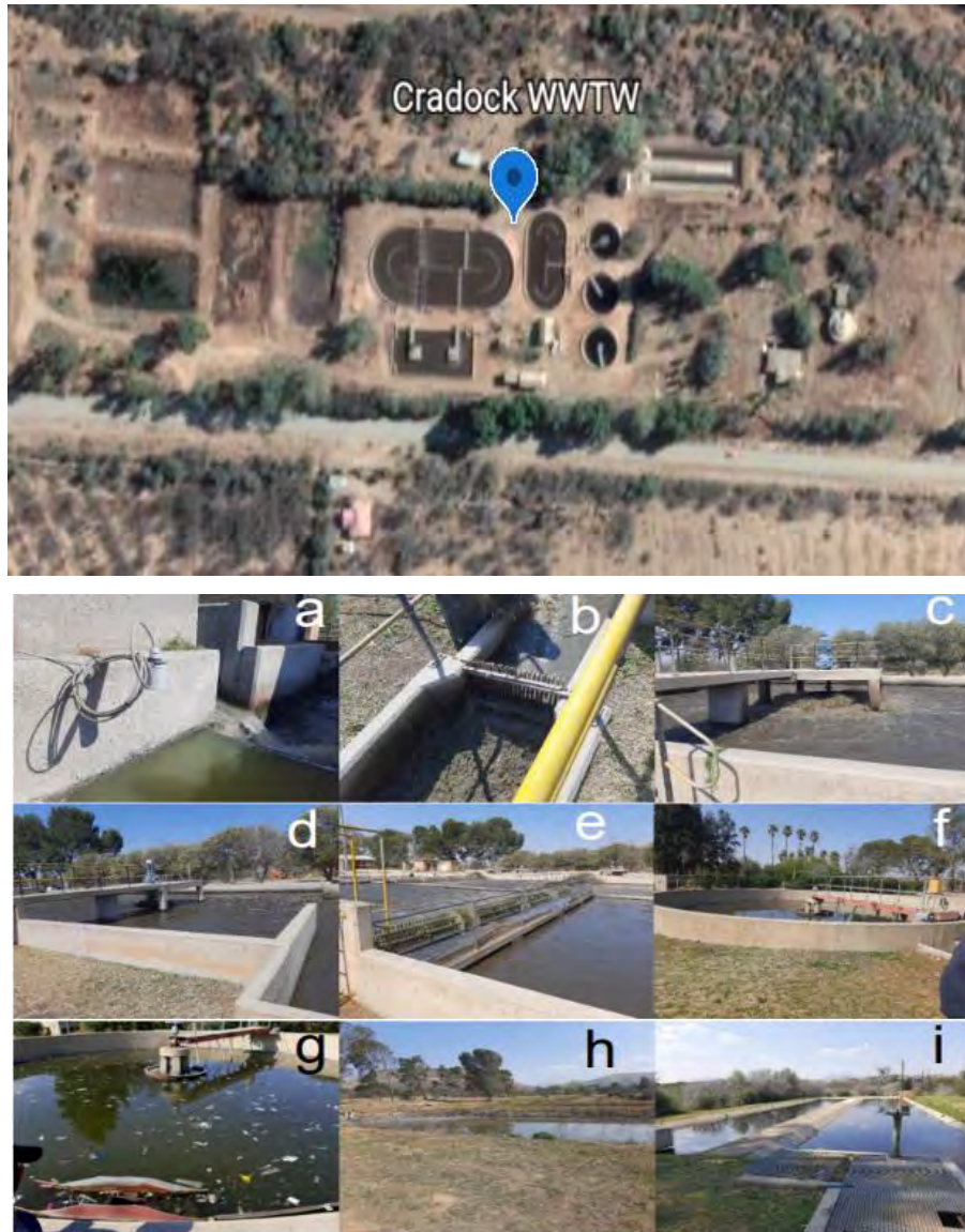
Figure 3.5 Cradock WWTW (top panel) and components of the process flow (bottom panel). a) wastewater flow into the WWTW; b) screening of the wastewater; c & d) grit chamber; e) aeration tanks lateral aerators; f) removal of excess bacteria in a sedimentation tank; g) clarification in Dortmund clarifiers; h) Landfill; i) Storage tanks for chlorinated wastewater before final treatment and discharge.
